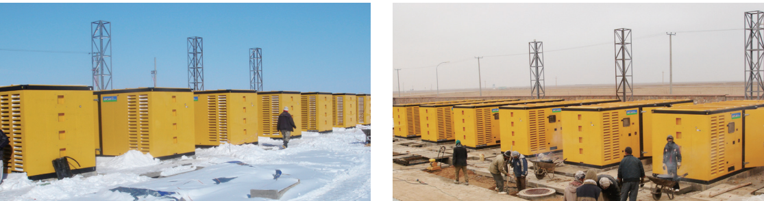
The Algerian state power company 20 units , 880KVA, 10KV container rites high voltage gensets runs weaver.
