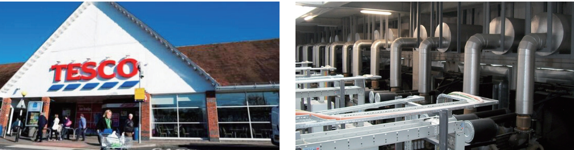
British Tesco supermarket , 31 units gensets , power involves 650KVA~1435KVA, the total capacity of 34065KVA.
