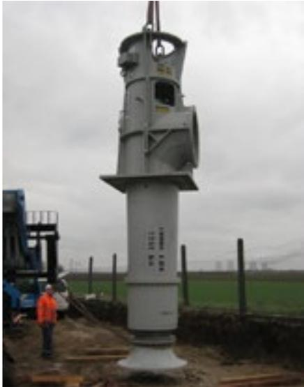
The transport of large flows requires large hydraulics and motors with the highest efficiency. Even a small increase in efficiency translates into considerable cost-savings. While well-approved submersible motors are available up to 700 KW, a wet pit column pump can offer unlimited motor power to reach theoretically unlimited flows.
